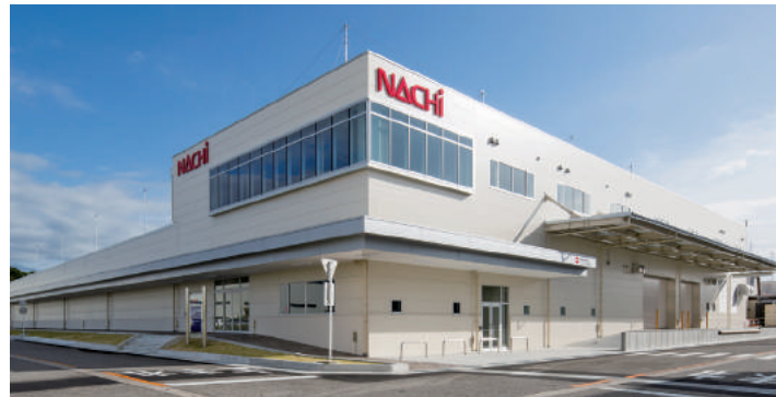
Automotive hydraulics factory 4 (completed November 2019)
