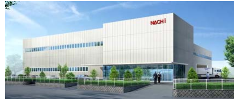
NACHI Engineering (April 2007 open)
