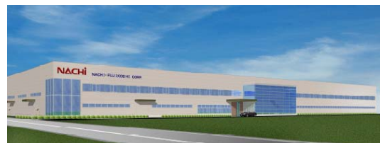
New Hydraulics Factory (Namerikawa groundbreaking, autumn 2007)
