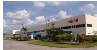
Thailand No. 3 Factory New Construction
