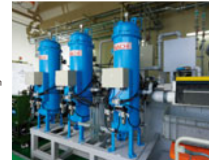
Centralized coolant equipment
