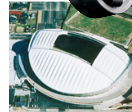
Bearings for opening/closing Stadium Domes
