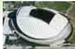
Moveable roof domes
