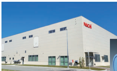
New hydraulic traveling motor plant
