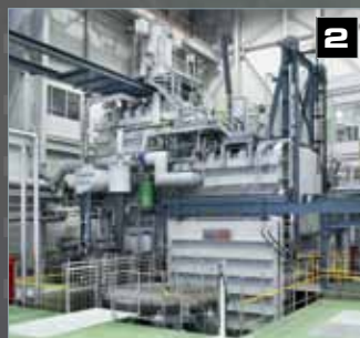
VIM furnace (vacuum induction melting) 3 tons
