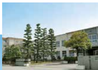
FUJIKOSHI Technical High School
